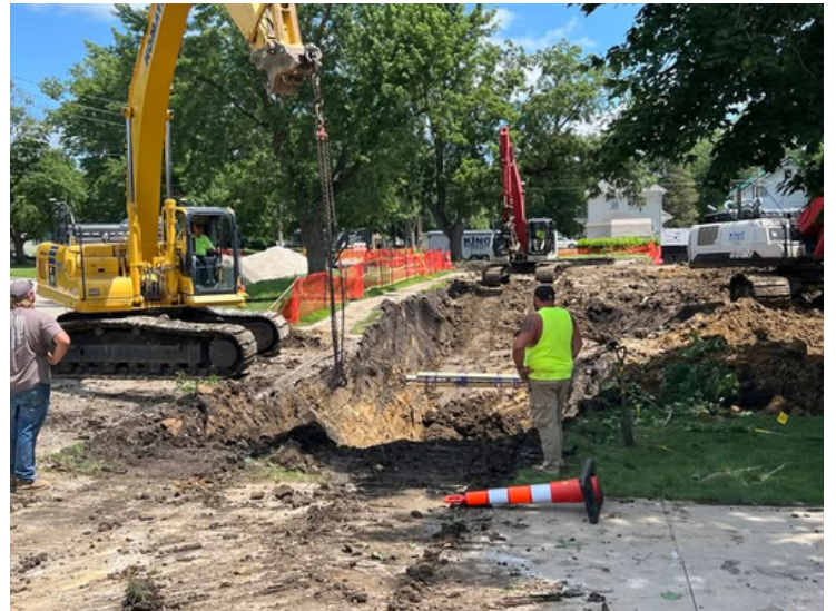
Construction began on three lift station replacements.
