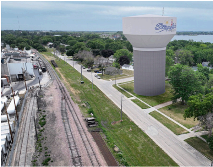
Construction neared completion on 1.5M gallon tower
