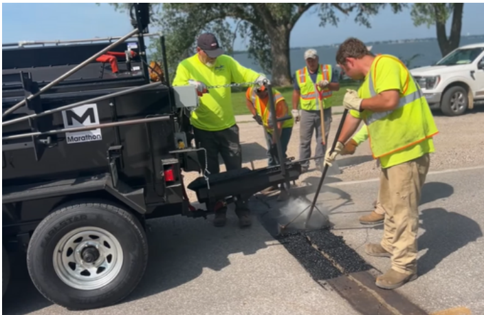
Streets repaired/resurfaced, new equipment added.
