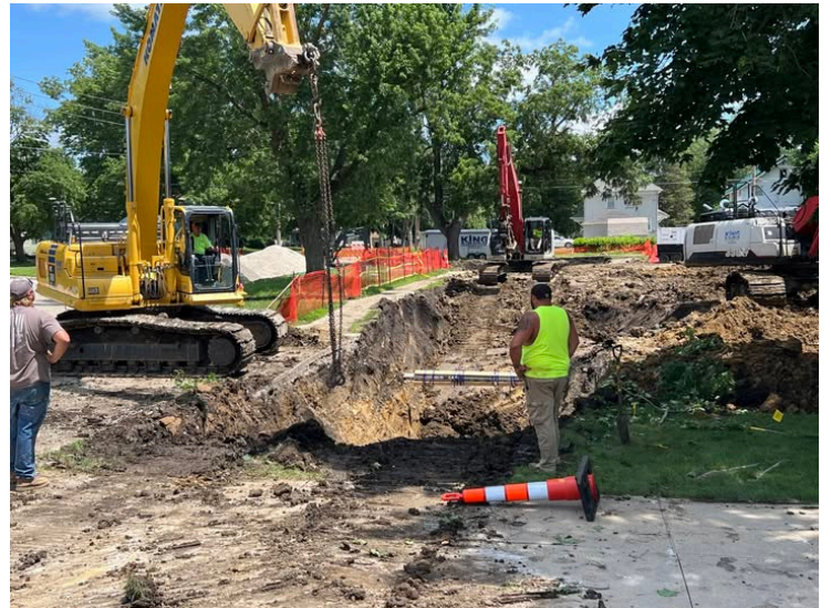
Three lift station replacements under construction.
