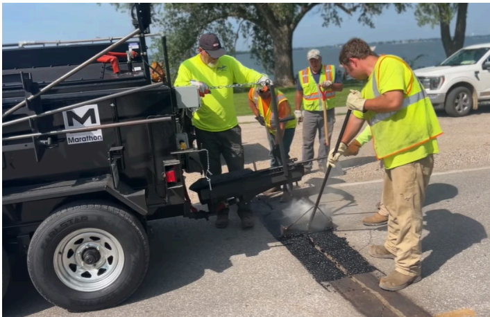
Streets resurfaced/repared, new equipment added
