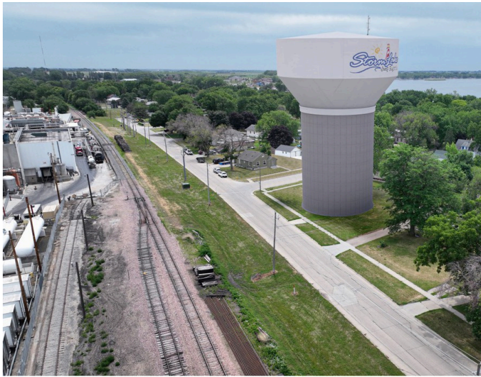
Construction nears completion on 1.5M gallon tower
