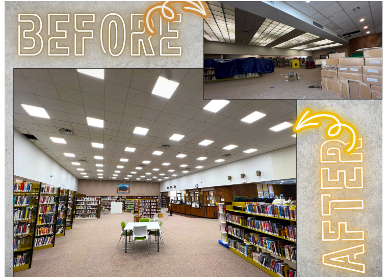
City buildings converted to energy-saving LED systems
