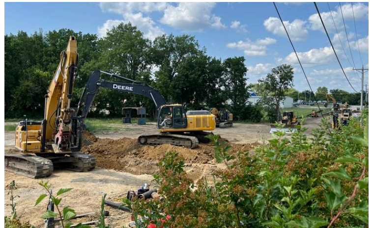
Memorial Road paving and infrastructure upgrades
