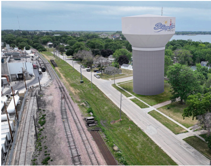
Construction for city's largest-ever water tower
