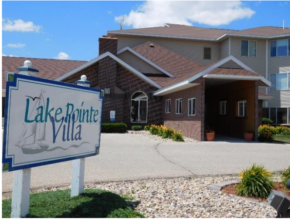
Methodist Manor – Lake Pointe Villa 1206 W 4 th St
