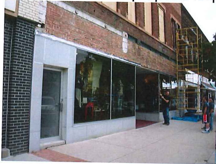
Shown with metal siding removed.
