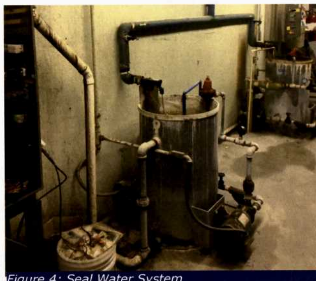
Figure 4: Seal Water System
