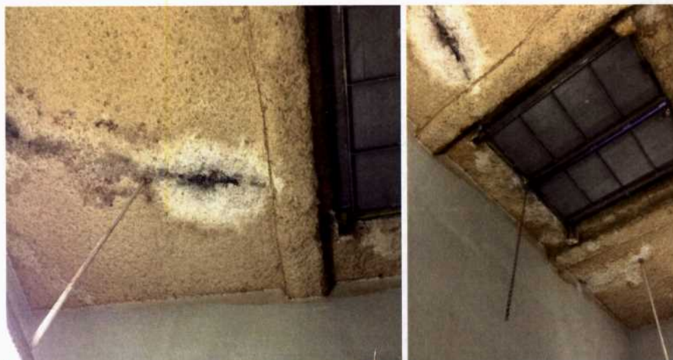
Figure 9: Electrical Room Ceiling
