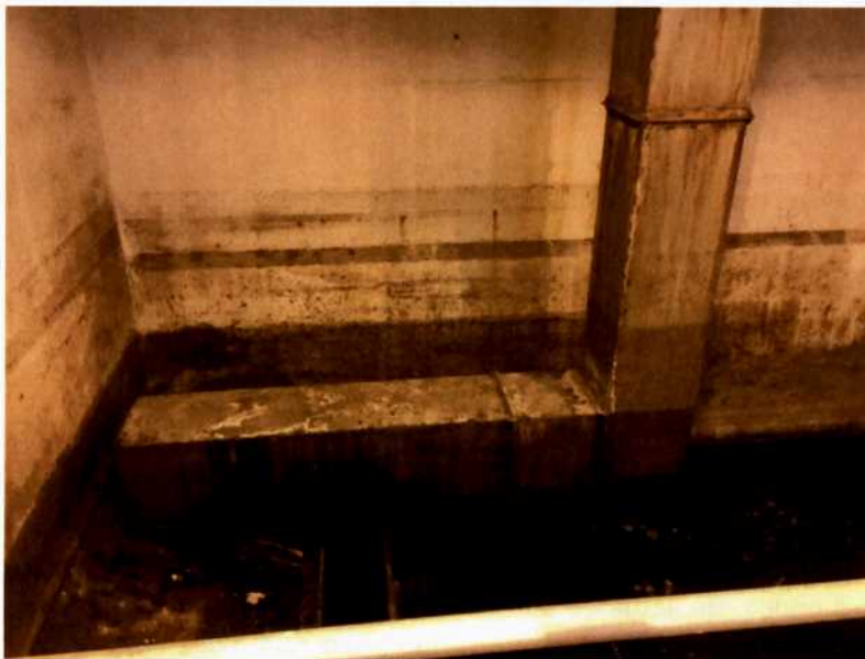
Figure 16: Headworks Chamber Exhaust Hood and Duct
