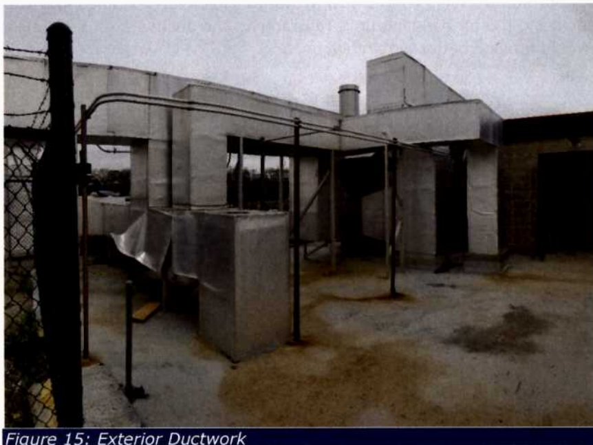
Figure 15: Exterior Ductwork
