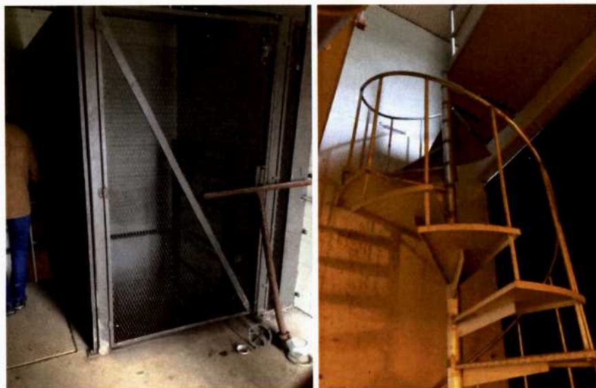
Figure 13: Elevator and Spiral Staircase
