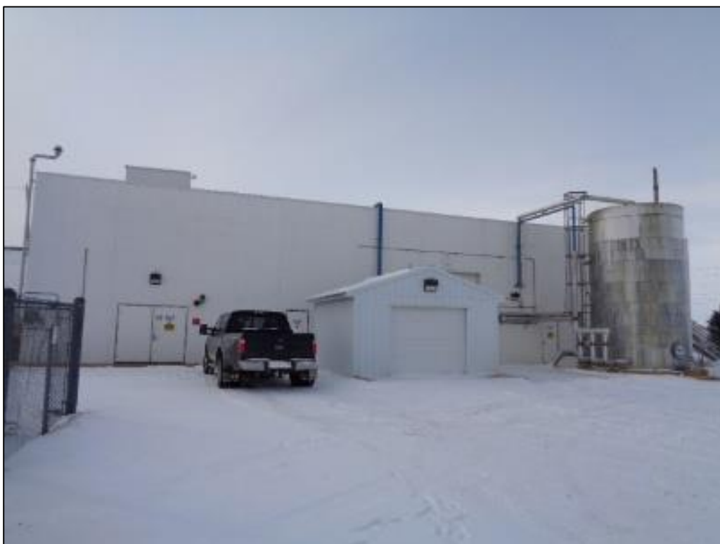
2000 Built Burner Building
