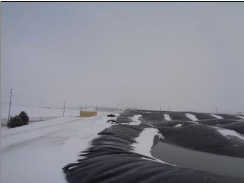
North Lagoons – Covered Anaerobic Lagoons
