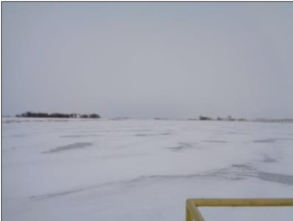
Effluent Final Lagoon - 6' Deep
