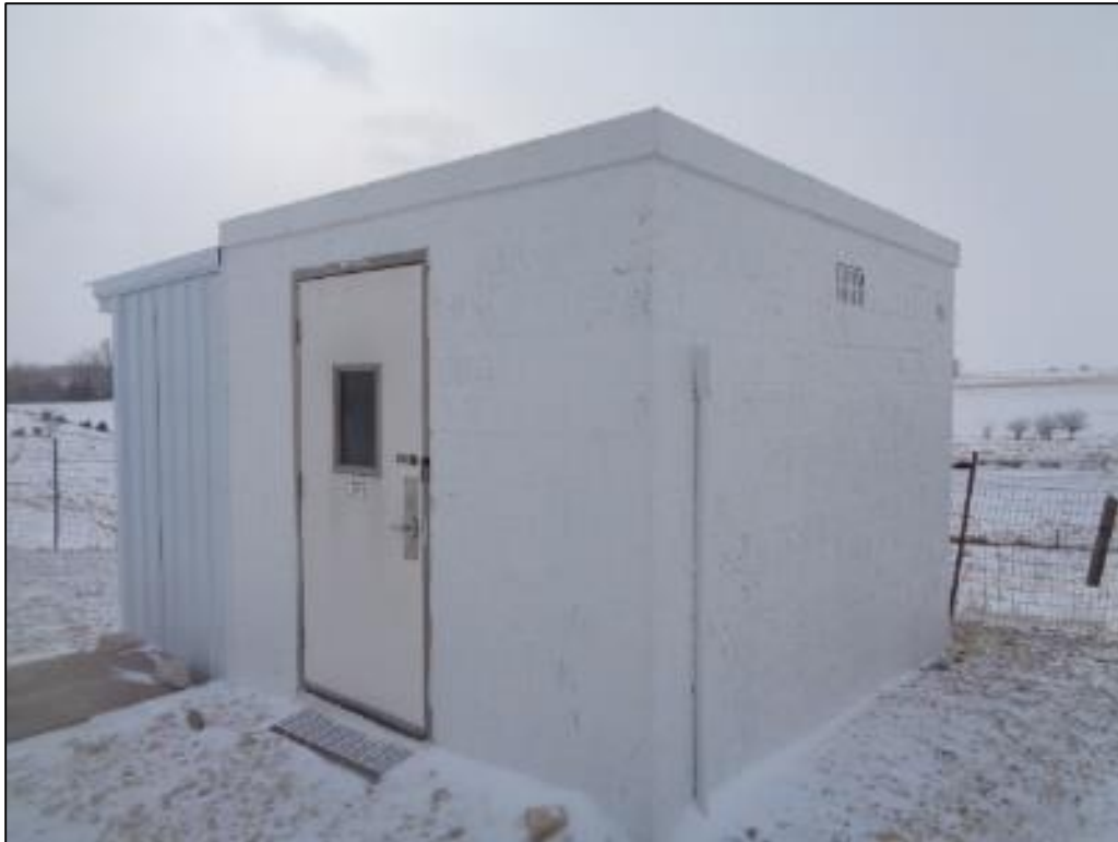
Shed on South Side of Property (Flow Meter, Sampler & Heater)
