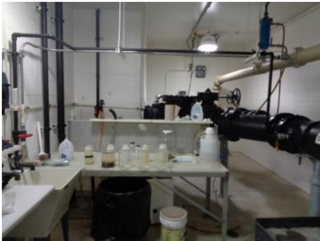
Pump & Lab Area For Concrete Pits
