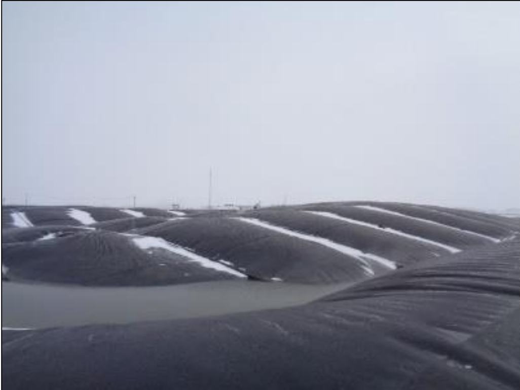
North Lagoons – Covered Anaerobic Lagoons
