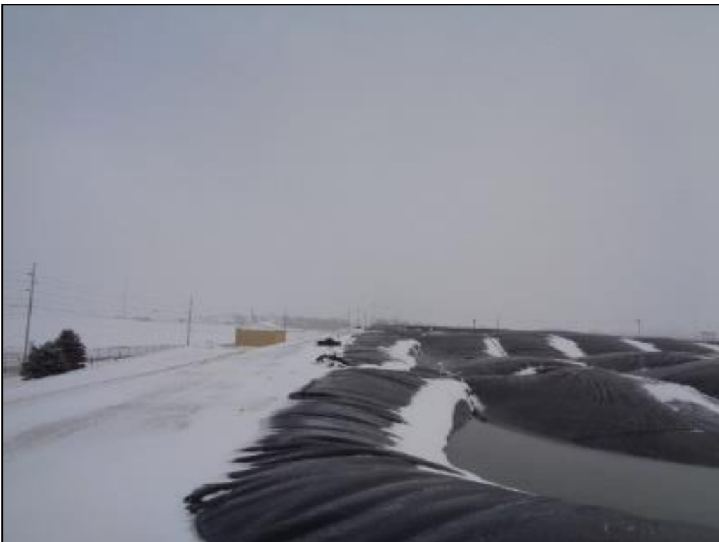
North Lagoons – Covered Anaerobic Lagoons
