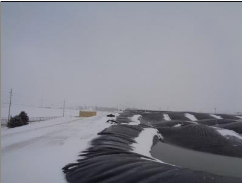
North Lagoons – Covered Anaerobic Lagoons
