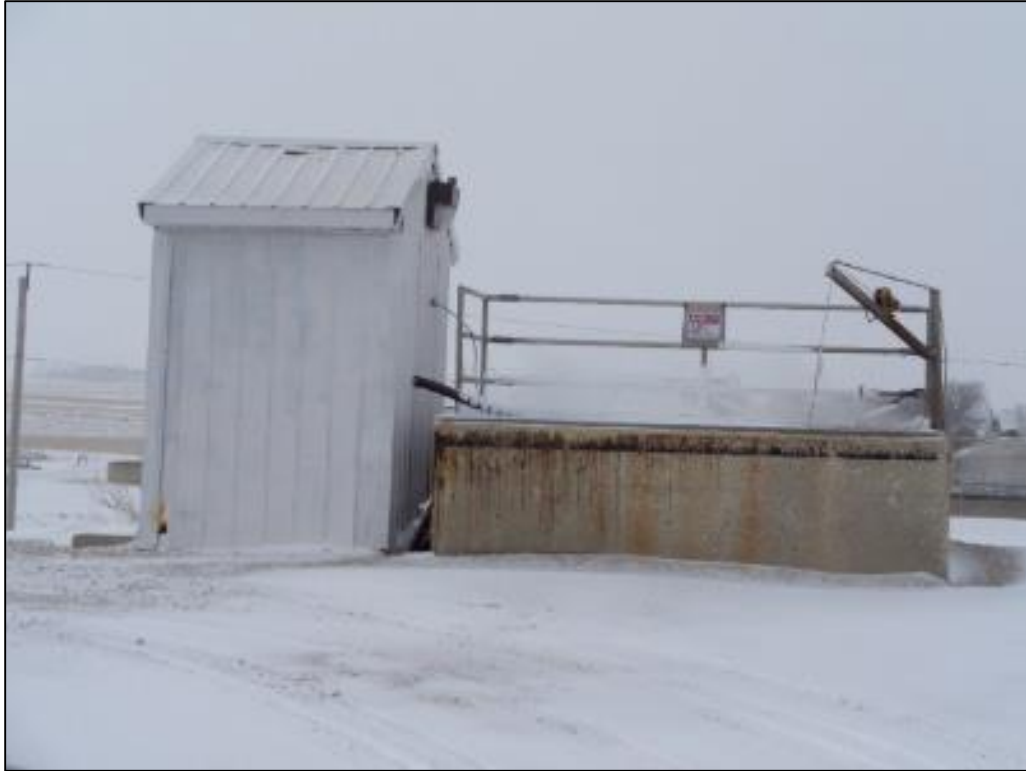
Influent Control Structure
