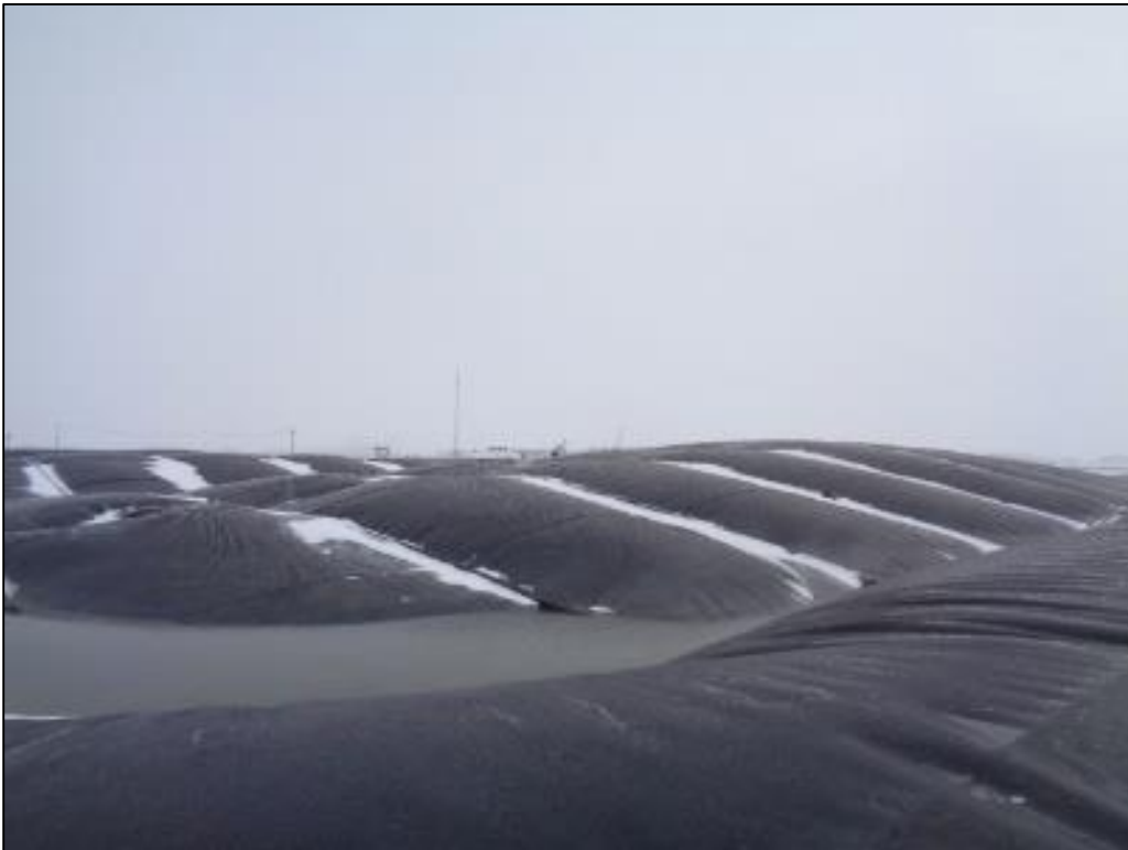
North Lagoons – Covered Anaerobic Lagoons
