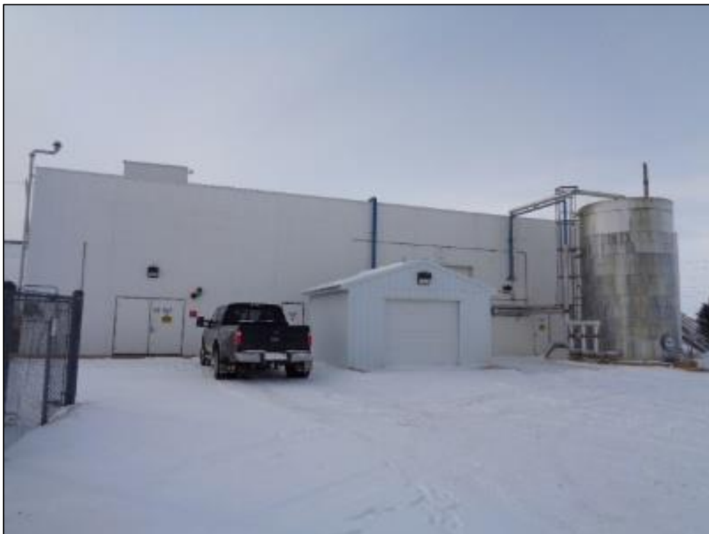
2000 Built Burner Building
