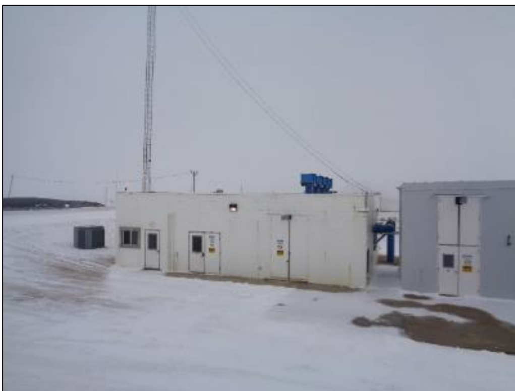
Office / Electrical / Chemical Storage (1966)
