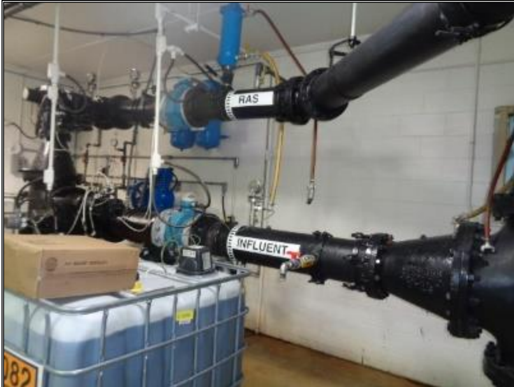
Pump Area For Concrete Pits
