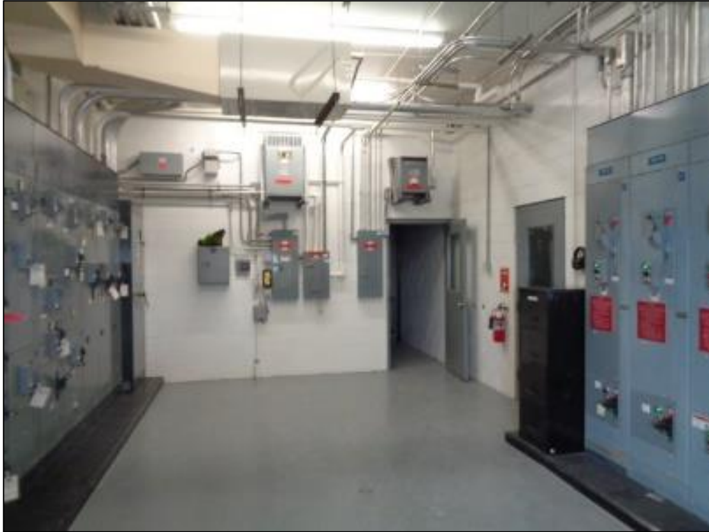
Electrical For Concrete Pits
