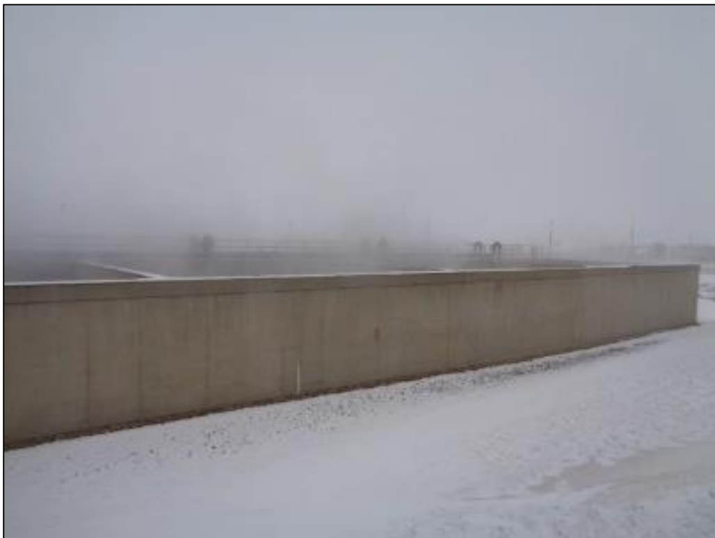
Concrete Pits – 18' Deep (2 Pits)
