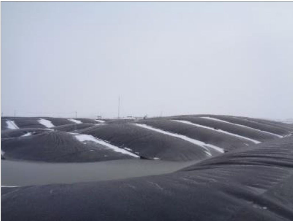
North Lagoons – Covered Anaerobic Lagoons
