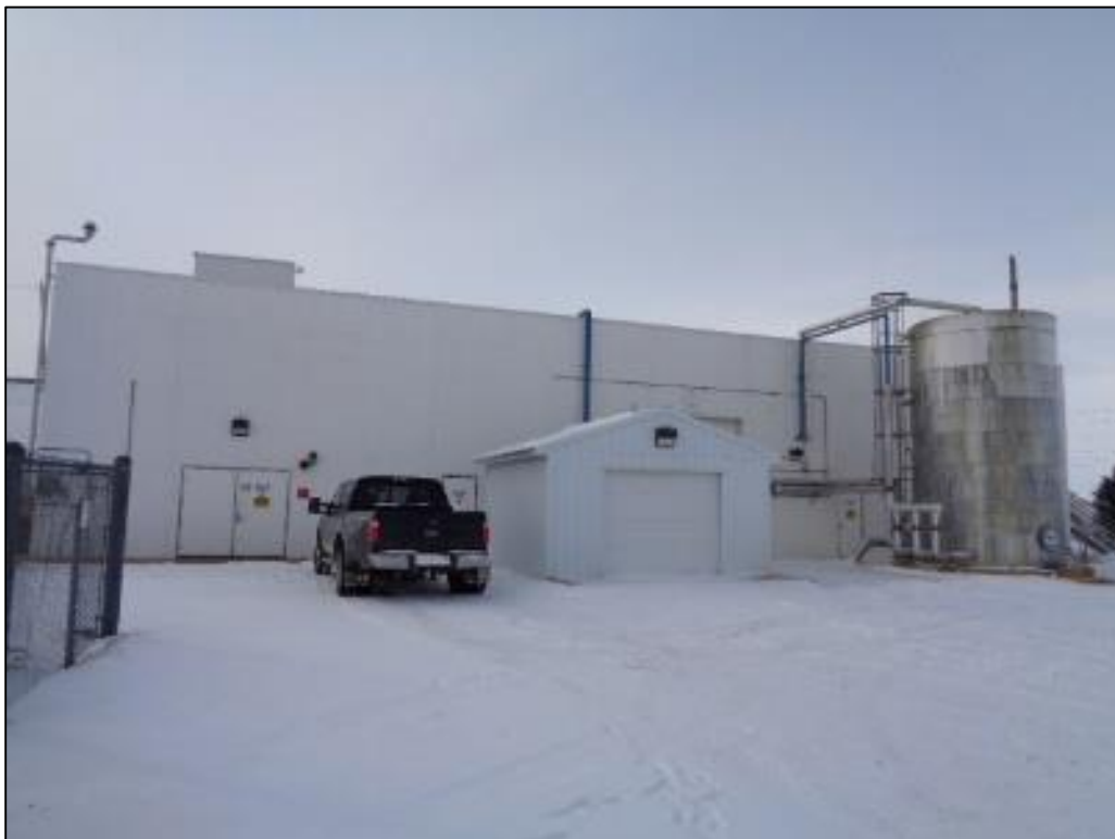
2000 Built Burner Building
